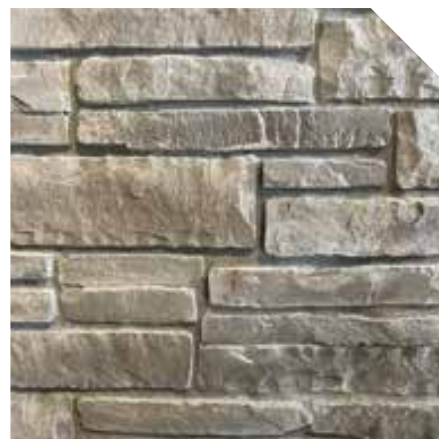
With hollow mortar joint
